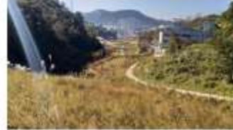
Area 5 Dam in upstream
