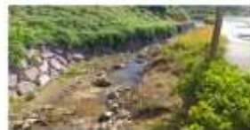
Bank protection with rock fill and vegetation
